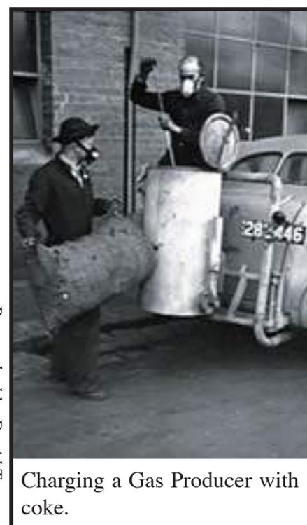
Charging a Gas Producer with coke.
