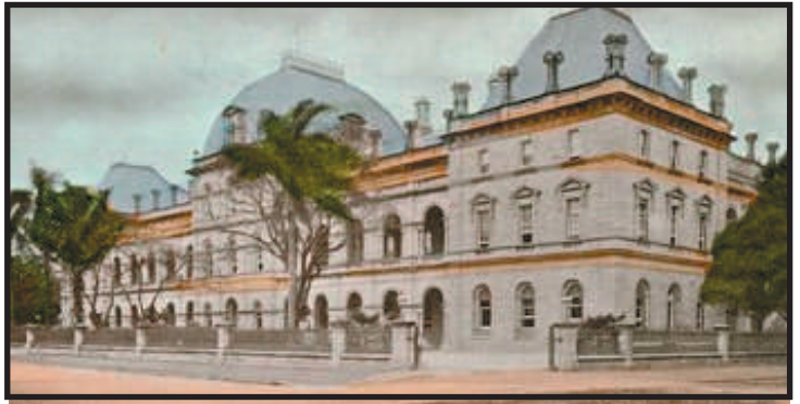
THE ADDITION OF COLONADES c1880s
