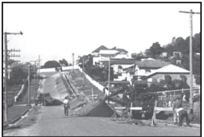
WORKERS DIGGING THE TRENCH FOR THE SEWERAGE CONNECTION, ANTILL STREET, WILSTON. EILDON HILL AT RHS. 1949
