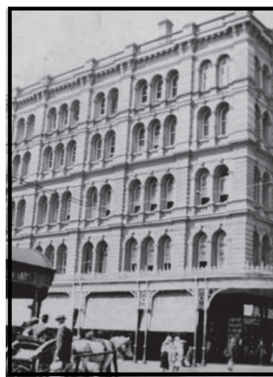
NEW COURIER BUILDING - CNR QUEEN & EDWARD STS.
